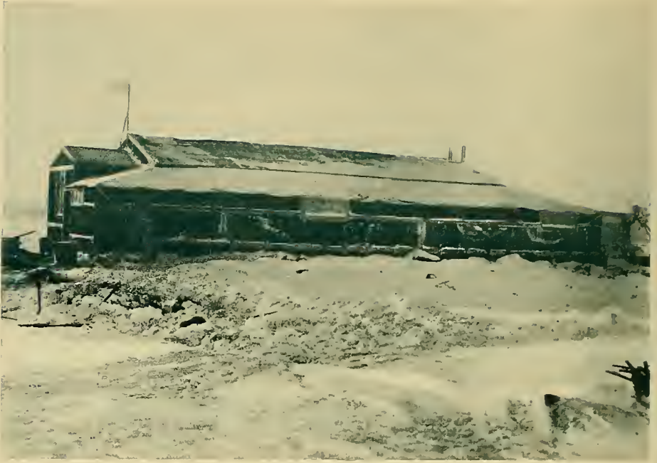
Rear view, showing warehouse
